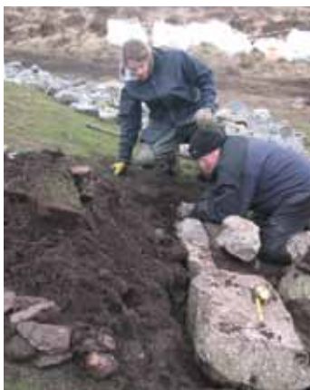
Contractors laying stone pitching
